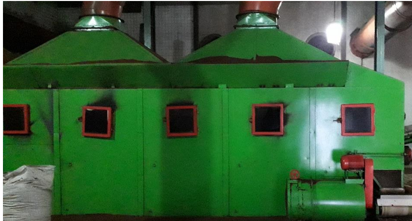
Gambar 1.16 Pengeringan ( Fluidized Bed Drying )
