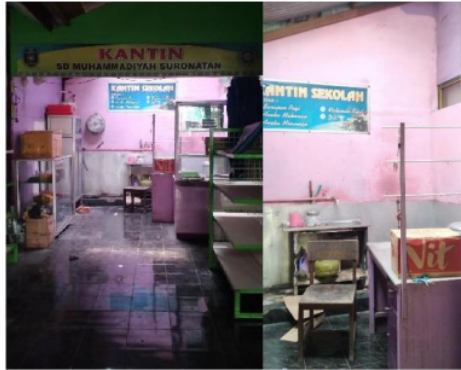
Figure 3. Condition of Canteen Processing Room
