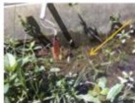
Figure 4. Installation of sensors
