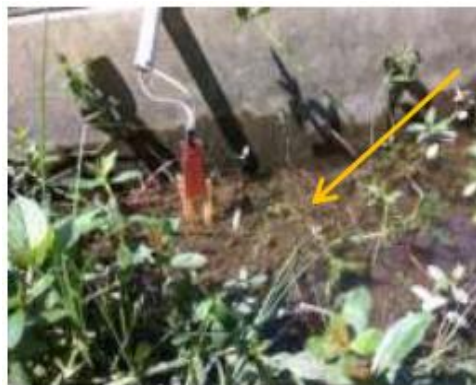
Figure 4. Installation of sensors
