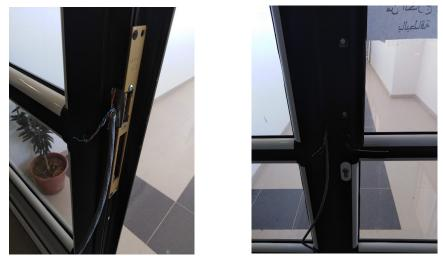
Fig. 12. The electric lock after integration of the proposed system
