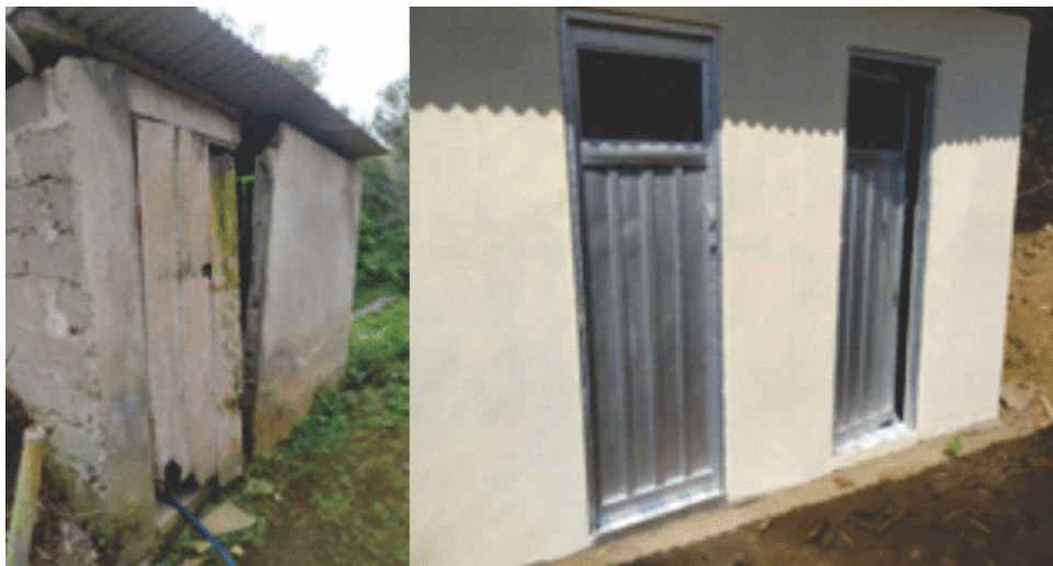
Figure 6. Before-after Toilet facilities
