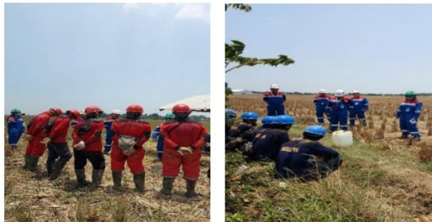
Gambar 16. Safety Talk Pekerja Drilling-Preloading 3D Kepuh
