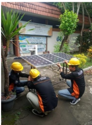
Fig. 6. Solar panel assembly
