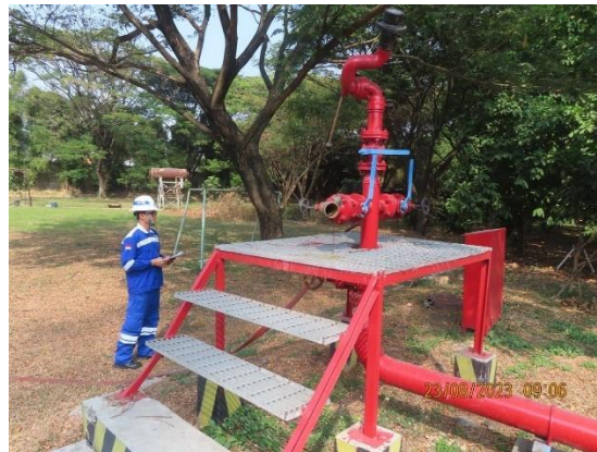
Gambar 15. Pengecekan Hydrant
