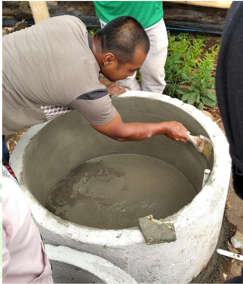
Gambar 5.5. Penambalan/pemolesan dinding buis beton
