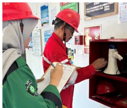
Gambar 21. Inspeksi Emergency Box
