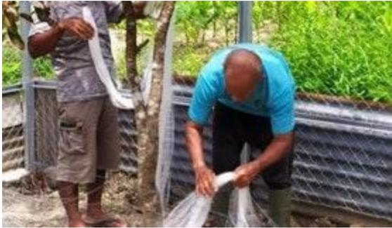
**Figure 4.** Installation of galvanized fence and paranet netting
