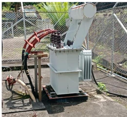
**Gambar 3.12.** *Trafo Auxiliary* PLTM Ndungga
