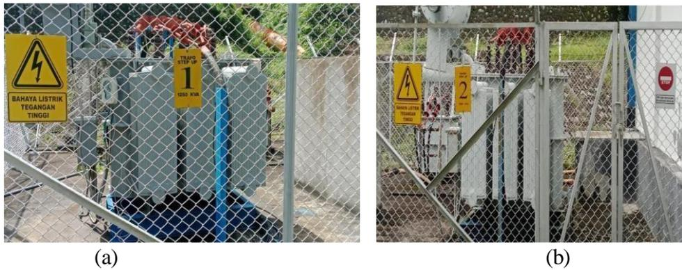
**Gambar 3.11.** (a) Trafo step-up unit 1 (b) Trafo step-up unit 2 PLTM Ndungga
